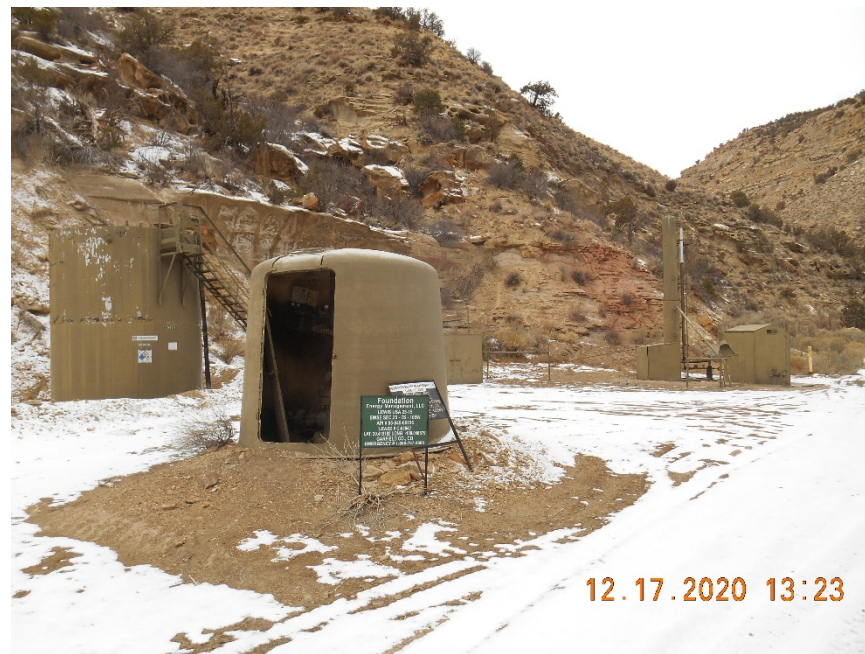
Wellhead inside housing with signs. Bradenhead plumbed to surface. CA completed.
