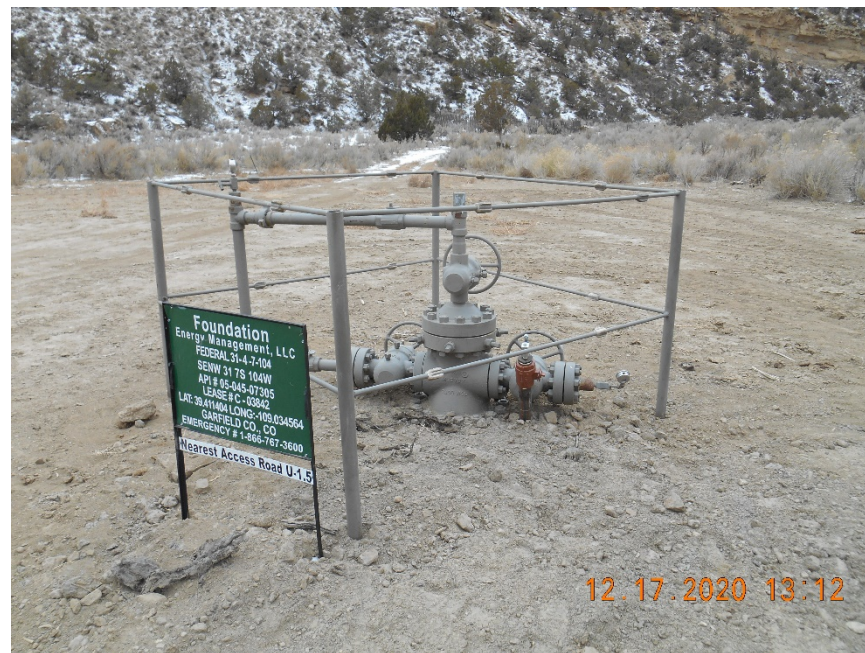
Wellhead with sign and fence. Bradenhead plumbed to surface. CA completed.
