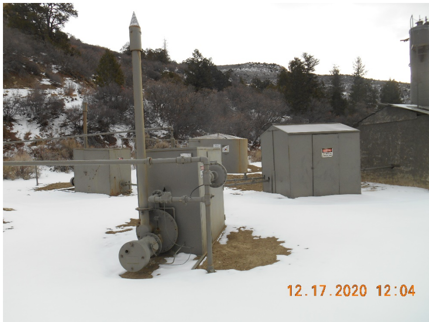
Separators, Dehydrator, Meter housing and Tank
