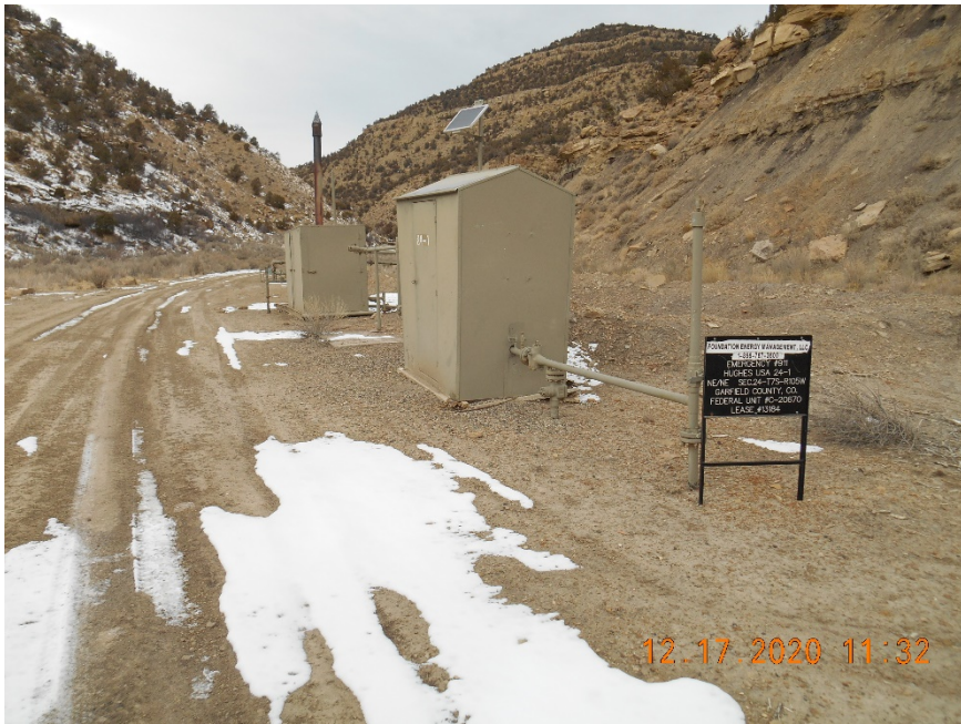
Location overview looking N.
