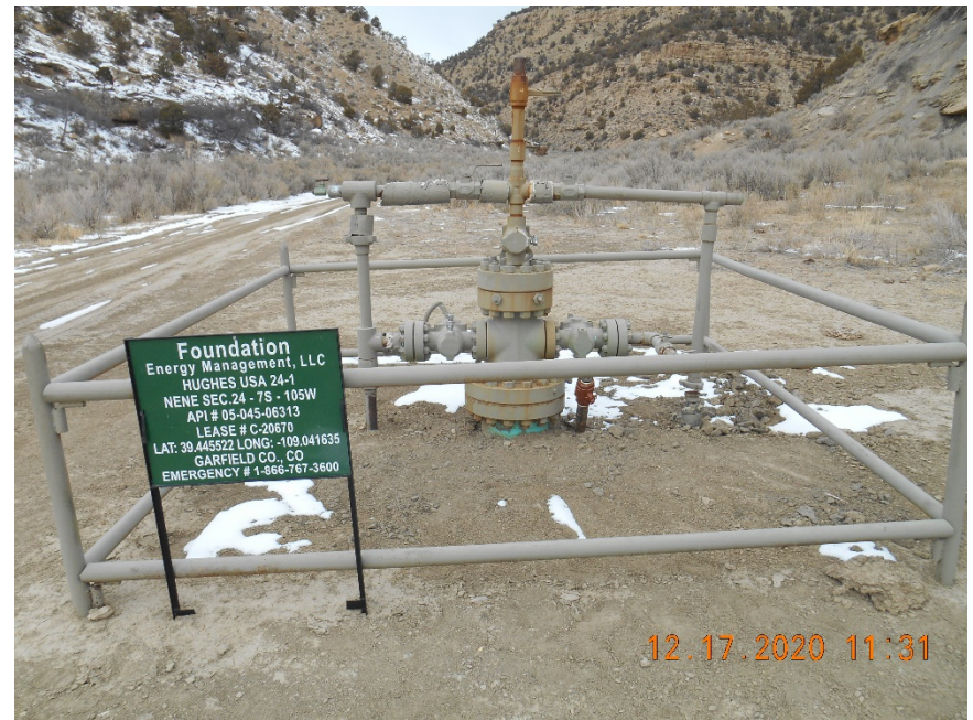
Wellhead with sign.
