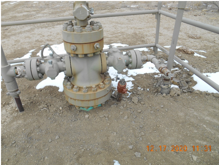
Bradenhead plumbed to surface. CA completed.
