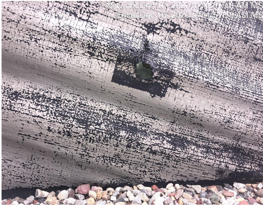
Photo #2478 Multiple holes in tank containment liner.
