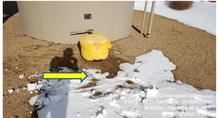
**Photo 1 Stained soil under load out line East tank**
