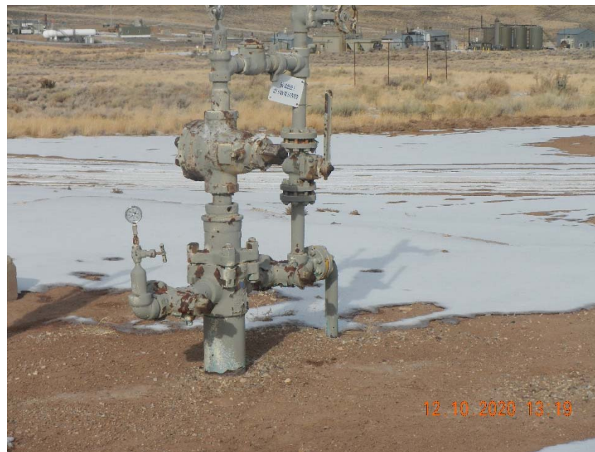
Photo 2. No bradenhead access apparent.
