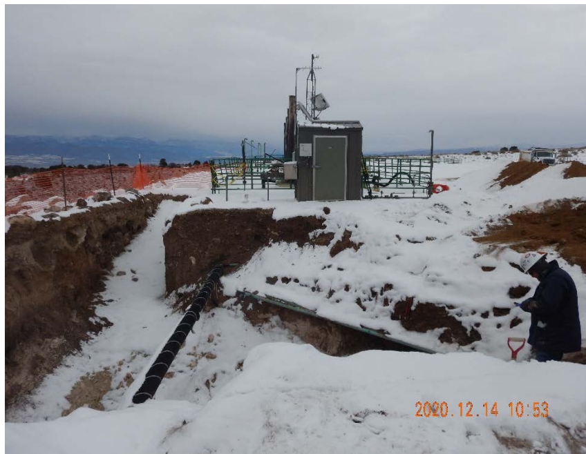
Photo #1 – View of open excavation from southwest. Note proximity of excavation to meter shed and separators as well as presence of multiple flowlines within excavation.
