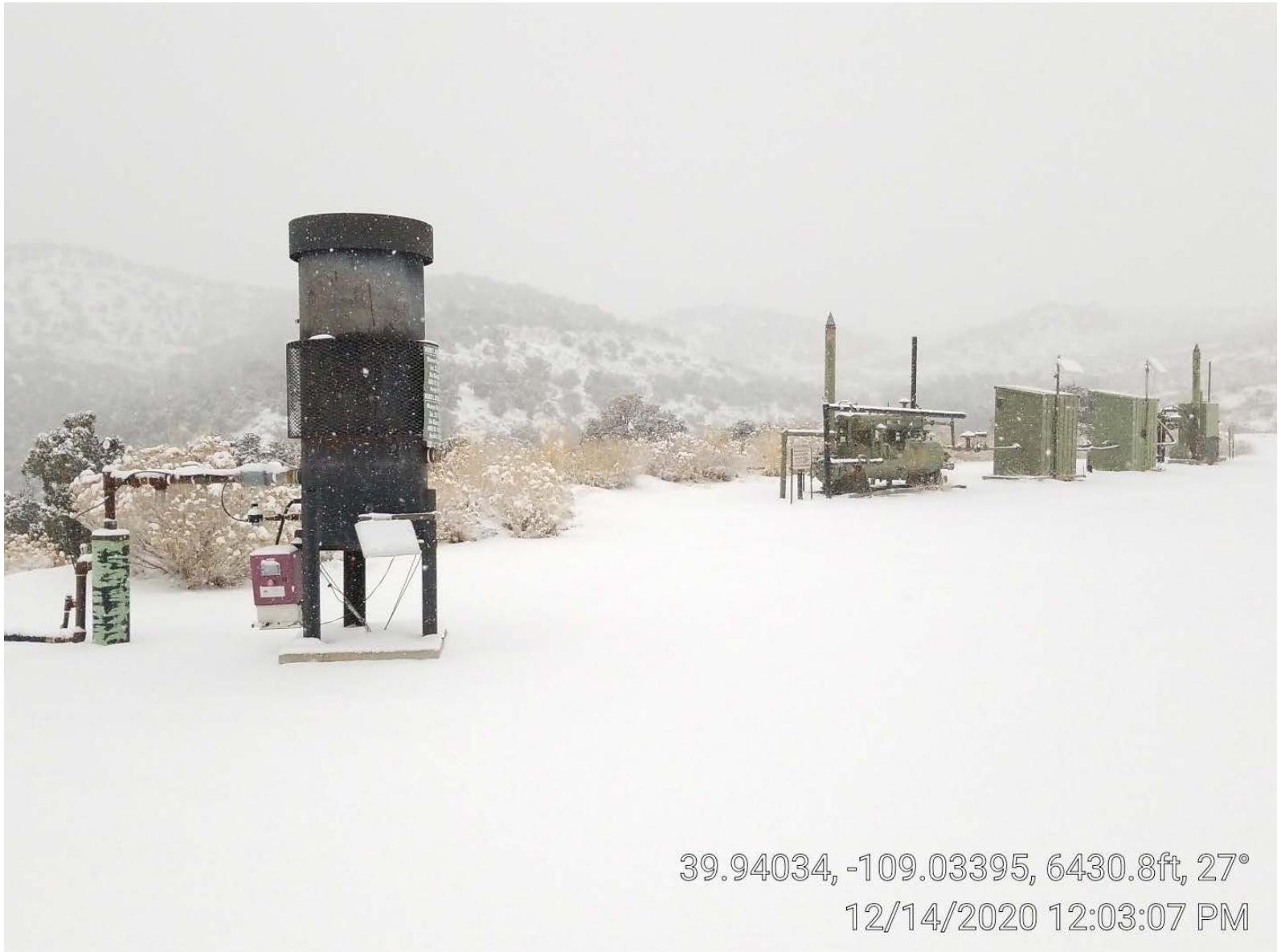
Photo 4. Combustor, meter buildings, separators.
