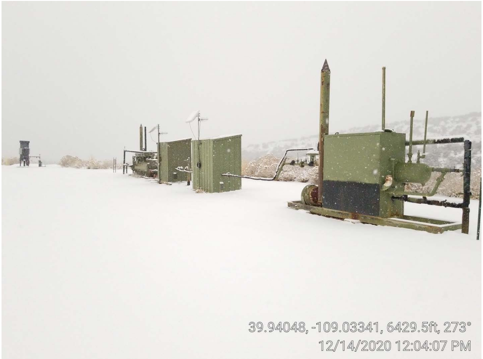
Photo 5. Separators, meter buildings, combustor.
