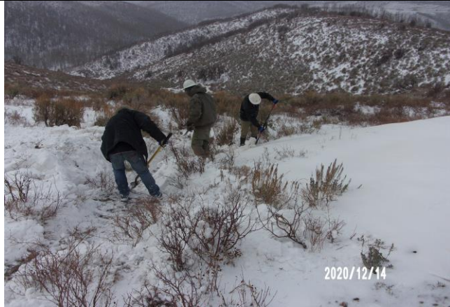
Wattle Installation on the C.C. 610-22-43
