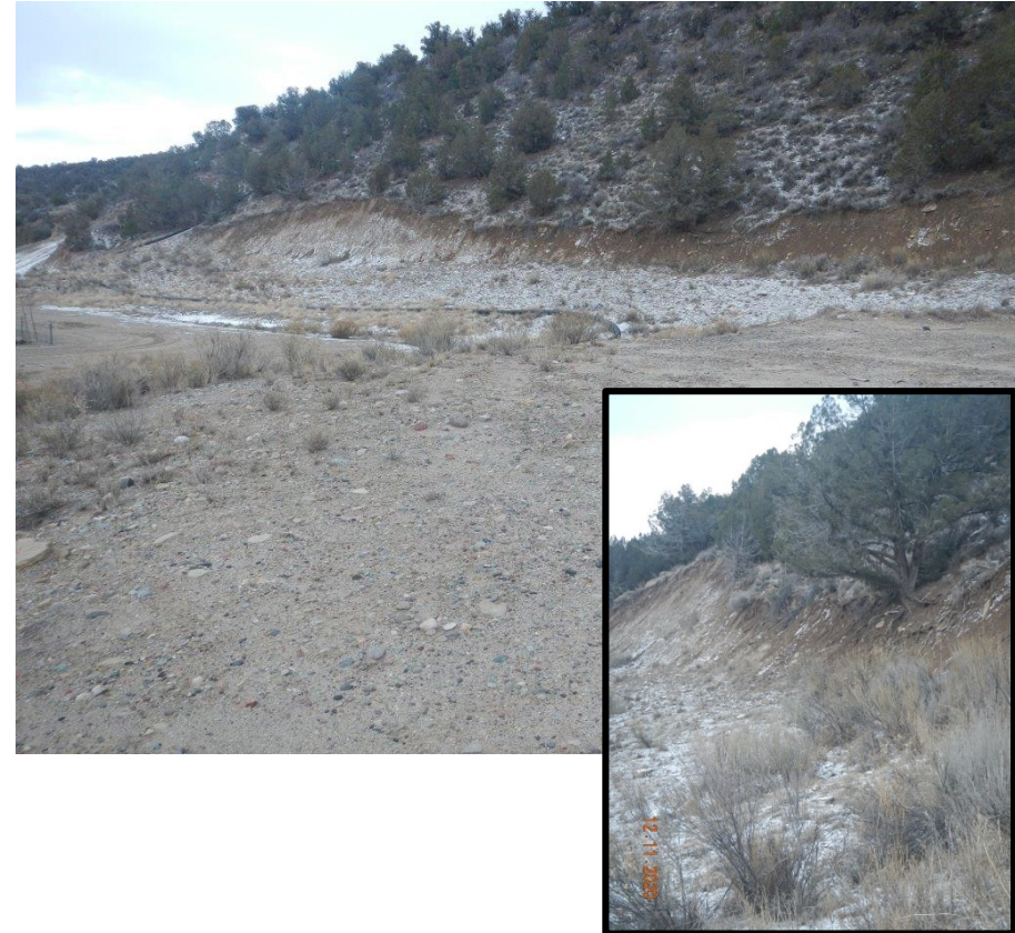
Photo#3: Cut slope, lower level Insert, detail of erosion
