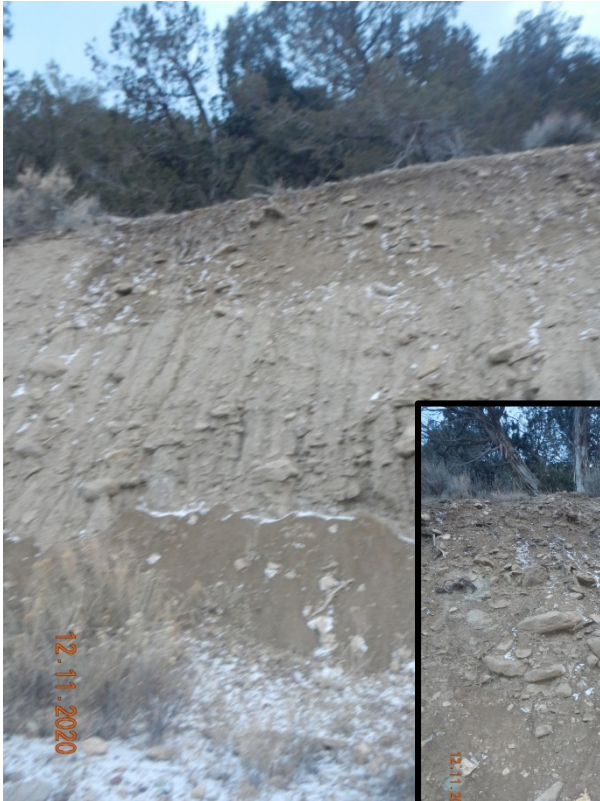
Photo#4: Erosion on cut slopes.
