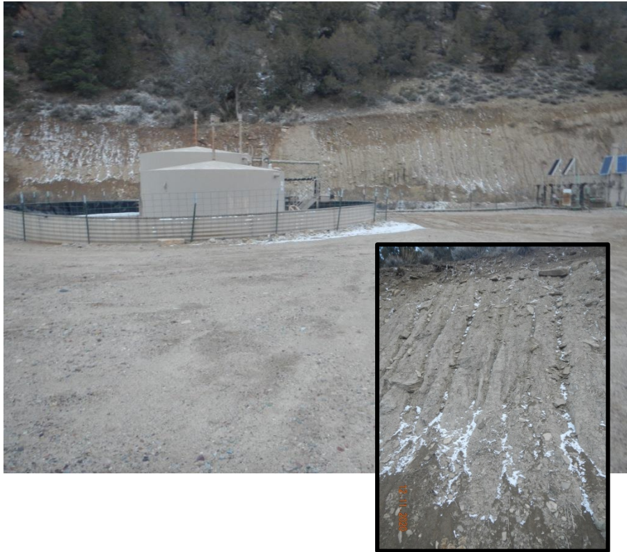
Photo#2: Cut slope, upper level. Insert, detail of erosion.
