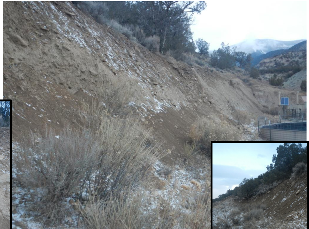
Photo#5: Erosion on cut slopes.
