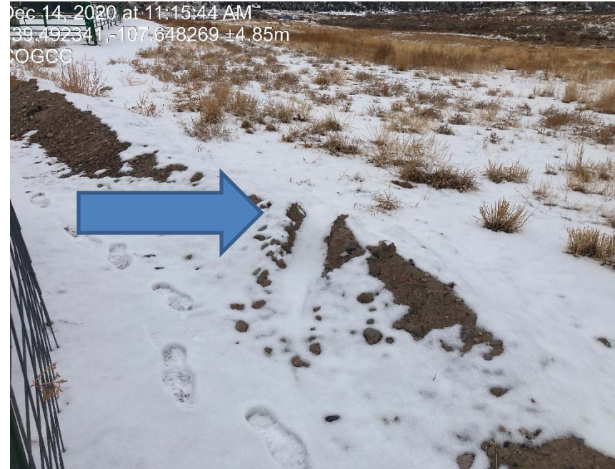
Berm next to combustor need maintained
