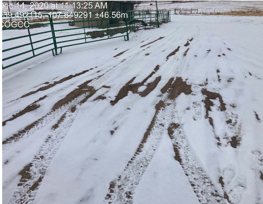
Lack of stabilization
