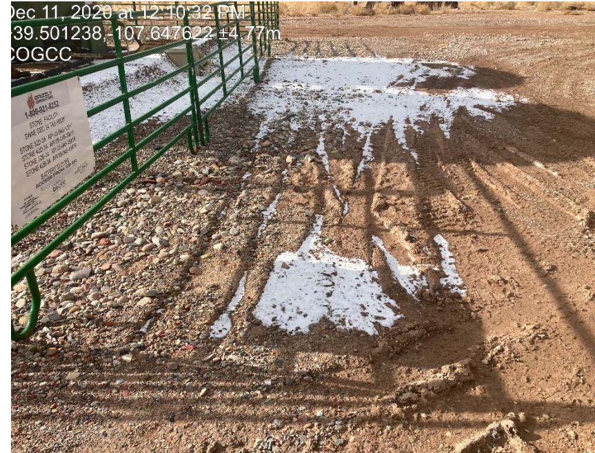
Lack of stabilization
