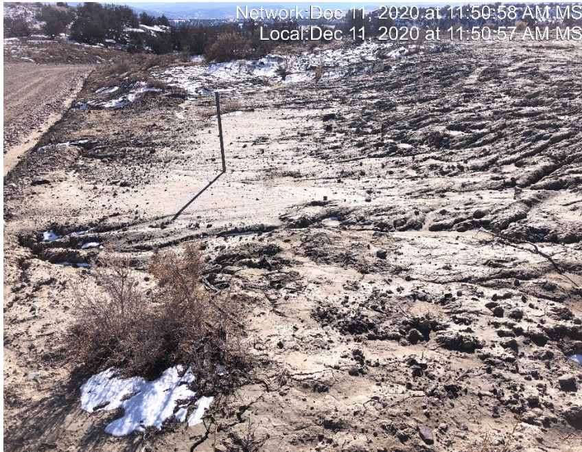
Photo #2457 Sediment migrating off of location and into access road ditch.
