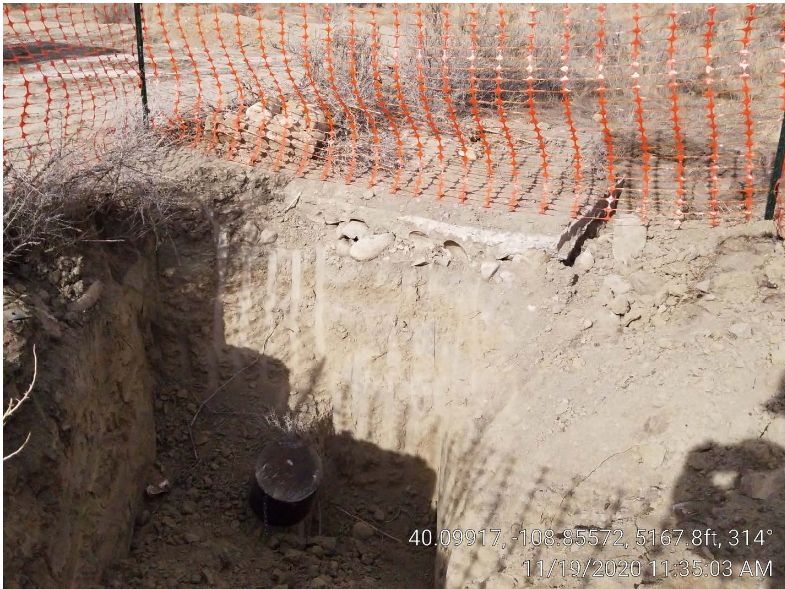
Photo 1. Well after casing cut off below ground level with hood on.
