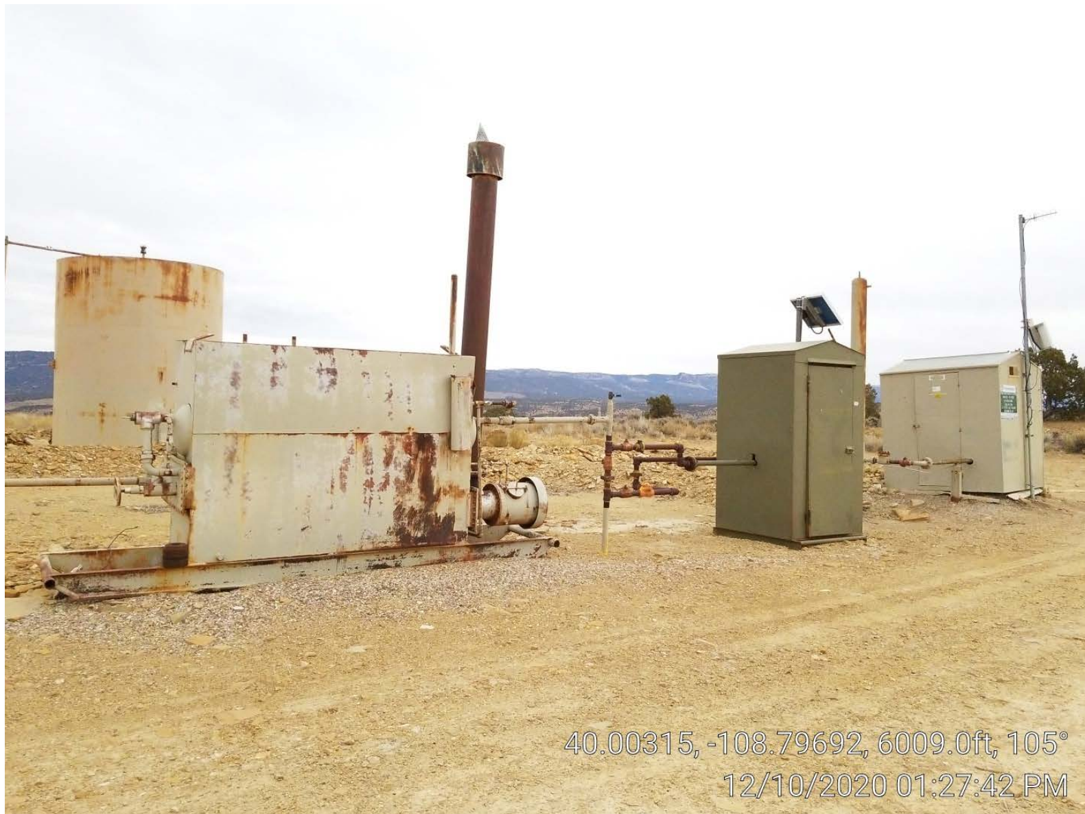
Photo 2. Tan, separator, meter buildings.
