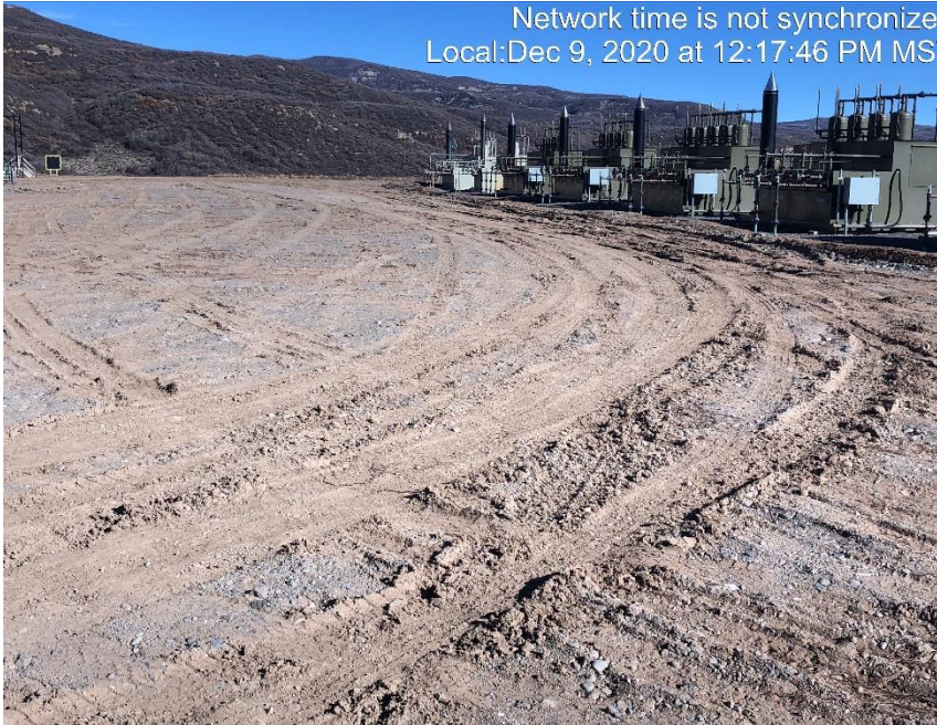
Photo #2432 Sediment is being transported off of location
