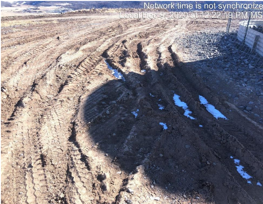
Photo #2436 Sediment is being transported off of location
