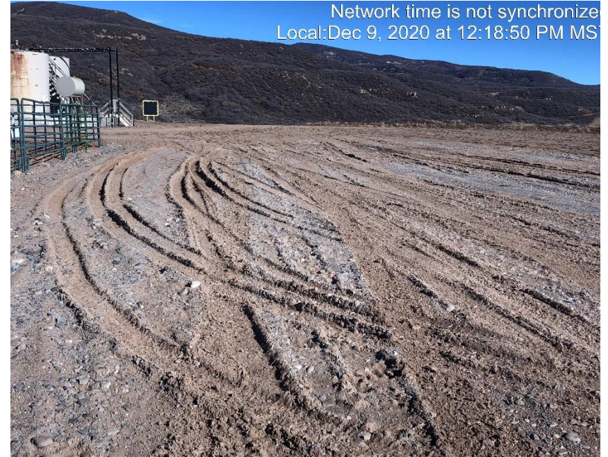
Photo #2433 Sediment is being transported off of location
