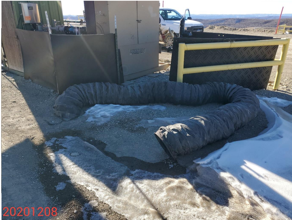
Photo 7: Photo shows equipment not stored in a workman-like manner.
