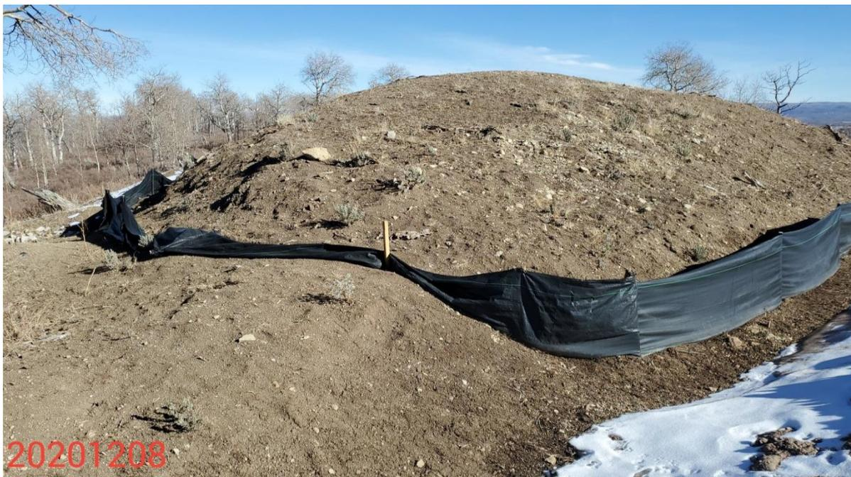
**Photo 6:** Photo taken from the northeast corner of the Location, facing northeast. Photo shows BMPs at the soil stockpile are missing or insufficient.
