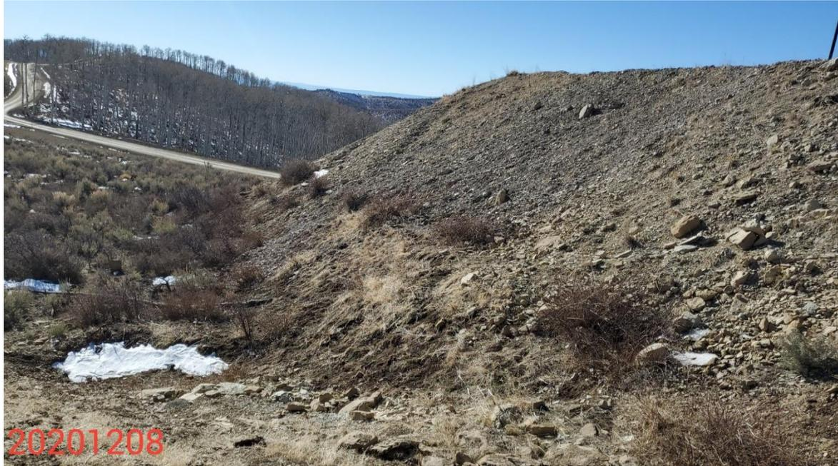
**Photo 16:** Photo taken from east end of the Location, facing south. Photo shows BMPs to stabilize/protect slopes, and prevent off-site sediment transport are missing, or insufficient
