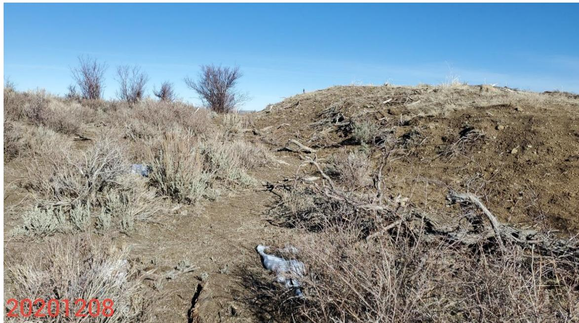
**Photo 15:** Photo taken from the southwest end of the Location, facing north. Photo shows BMPs at the soil stockpile are missing or insufficient.
