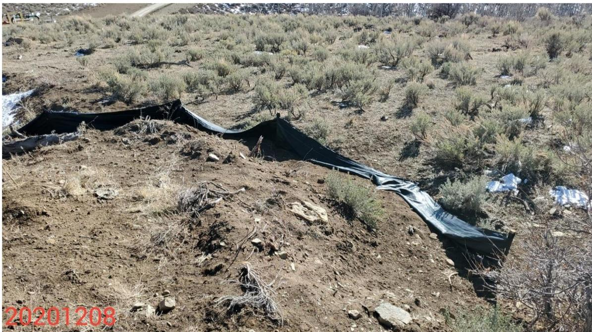
**Photo 14:** Photo taken from the southwest end of the Location, facing south. Photo shows BMPs at the soil stockpile are missing or insufficient.
