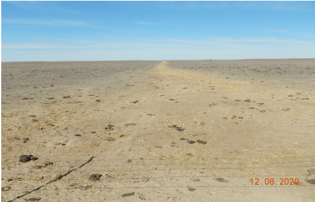
Photo 1. Facing north toward the access road. The road has been reclaimed and temporarily stabilized with straw mulch. It appears livestock have been utilizing the area near the fenceline and reclaimed road.
