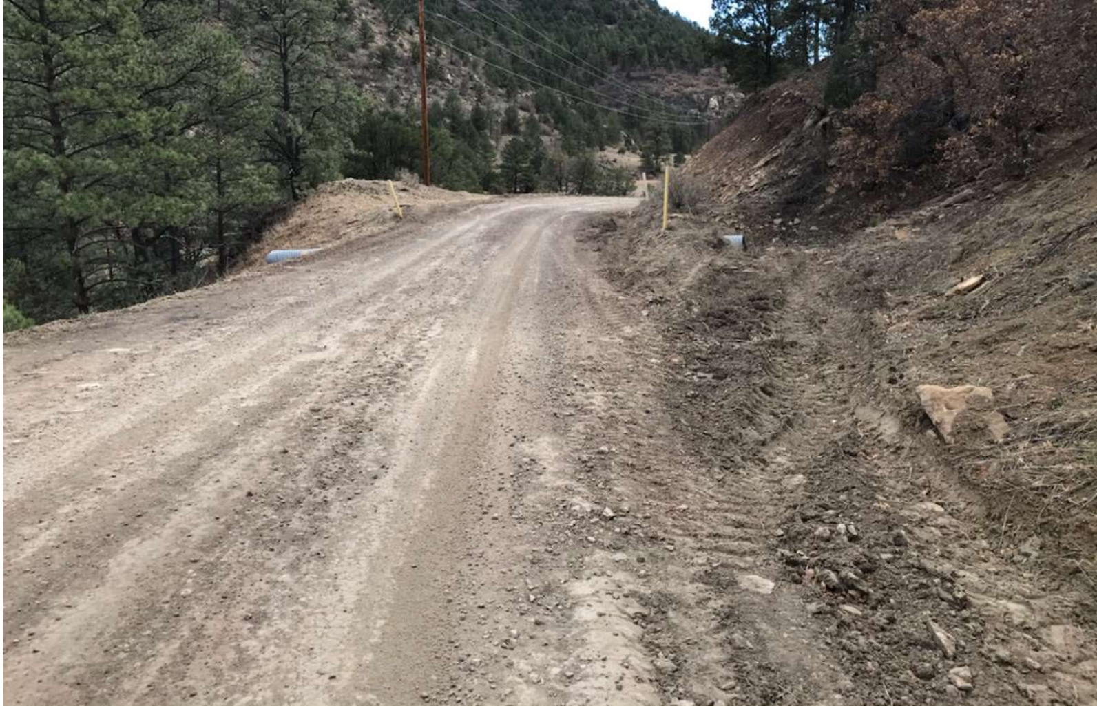
PHOTO 1: THE BAR DITCH WAS DOMINATED TO DIRECT SURFACE RUN OFF TO THE CULVERT INLET.
