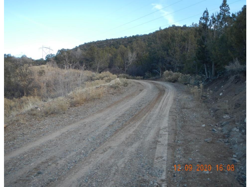
Ruts on access road.
