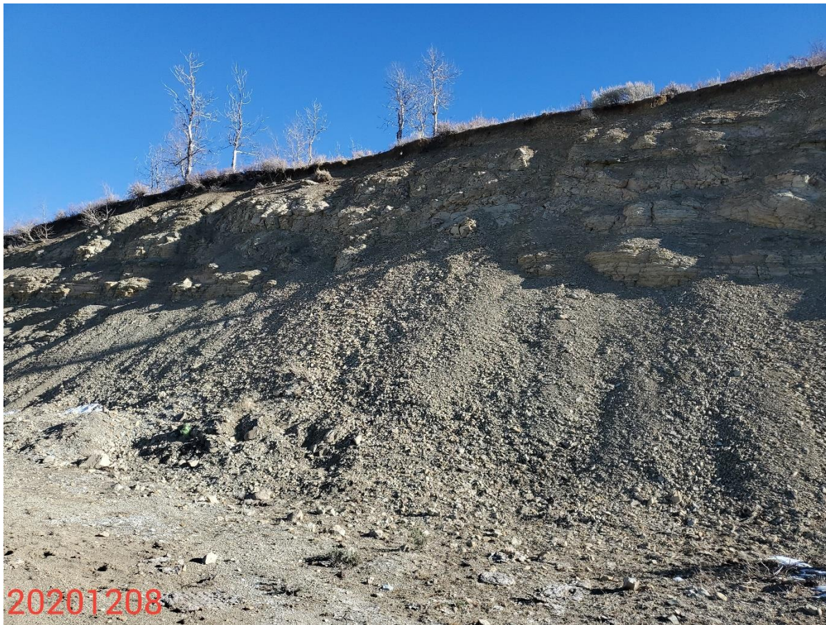
Photo 5: Photo taken from the east end of the Location, facing northeast. Photo shows BMPs to stabilize the cut slopes of the Location are missing, or insufficient.
