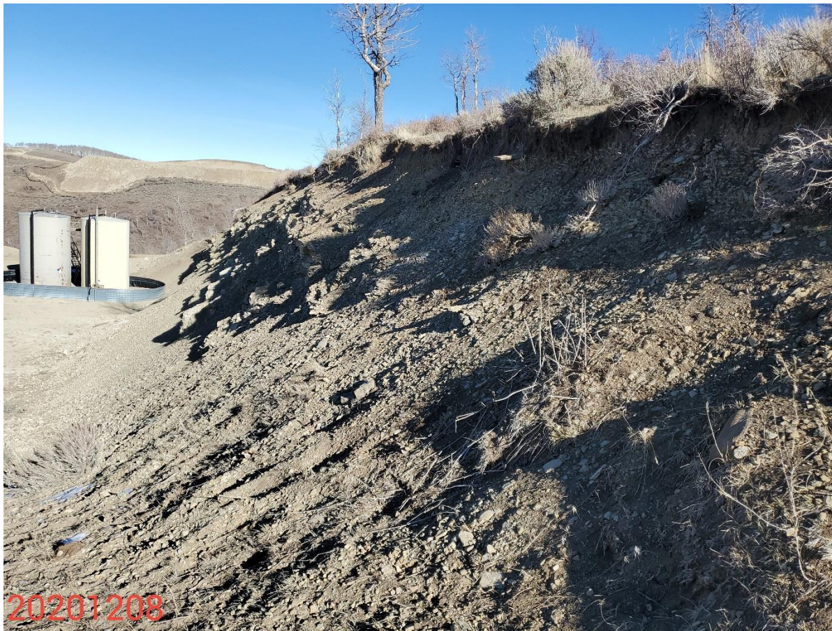
Photo 4: Photo taken from the southeast end of the Location, facing north. Photo shows BMPs to stabilize the cut slopes of the Location are missing, or insufficient.
