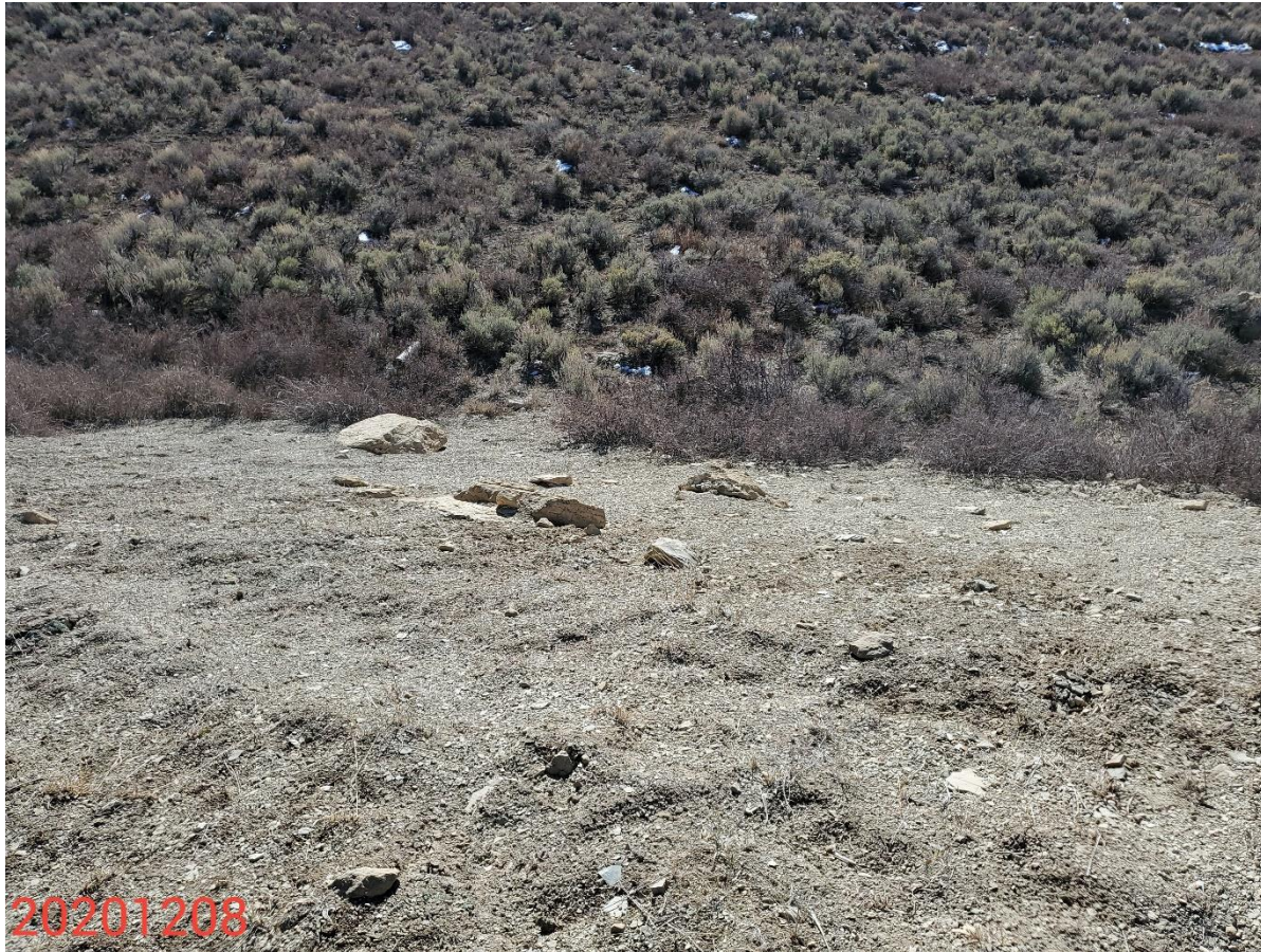
Photo 6: Photo taken from the south end of the Location, facing south. Photo shows BMPs to stabilize/protect the fill slopes, and prevent off-site sediment transport are missing or insufficient.
