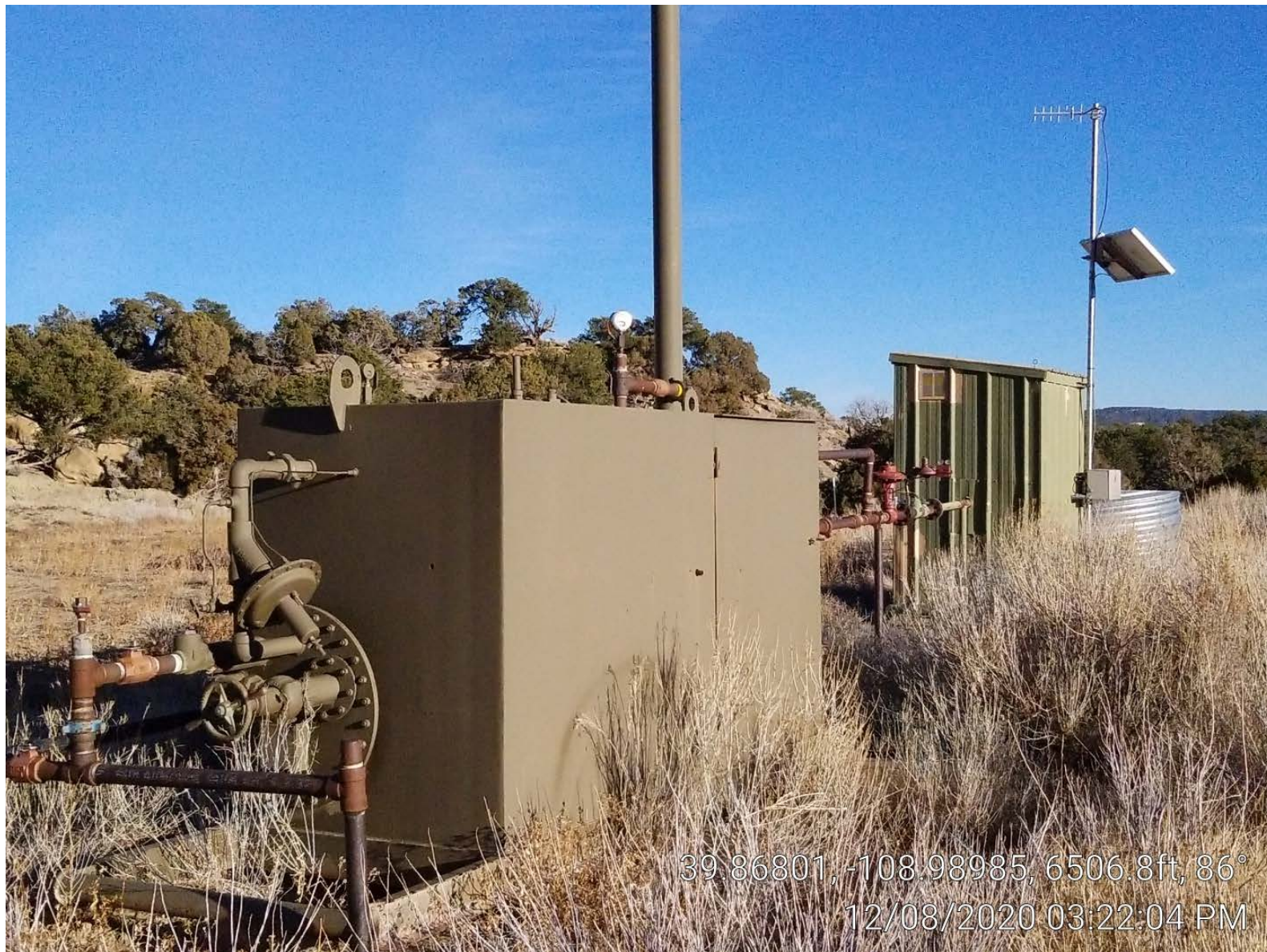
Photo 3. Separator, meter building.
