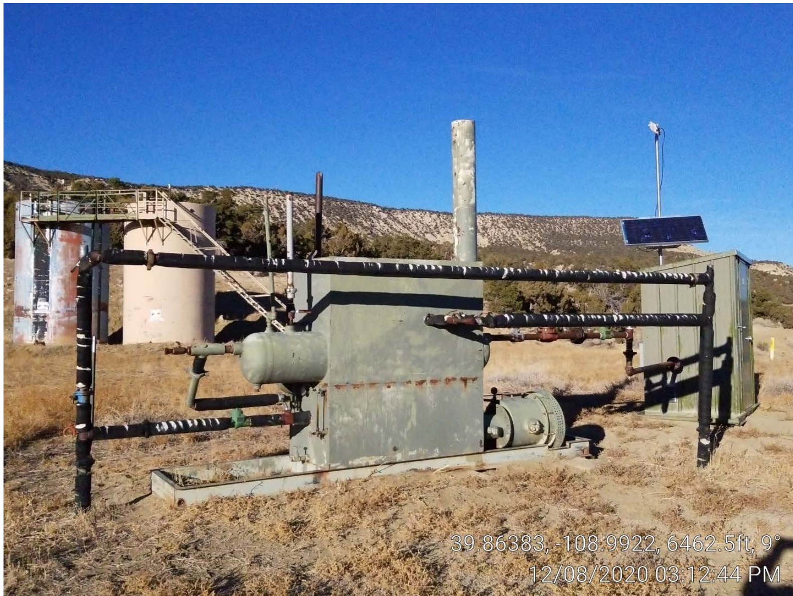
Photo 6. Tanks, separator, meter building.
