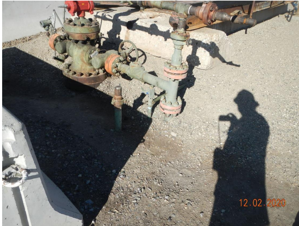
Unused and unmarked flowline riser
