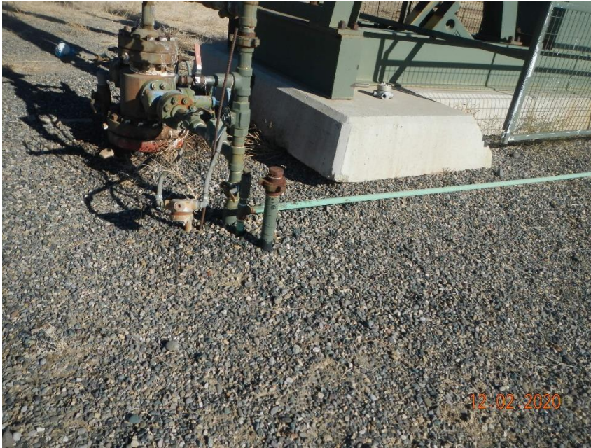
Unused and unmarked flowline riser
