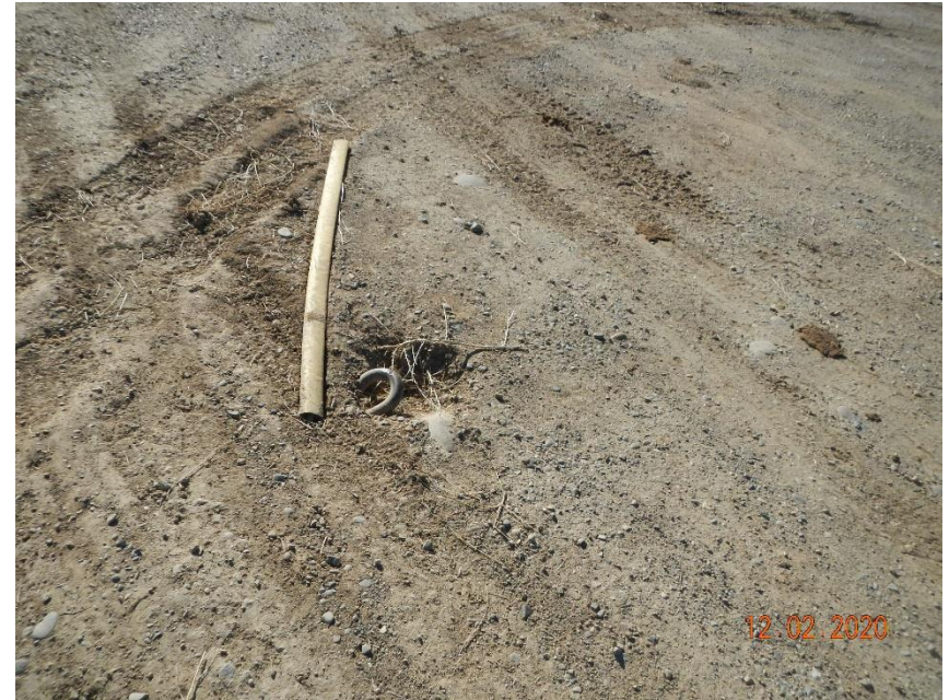
Most of rig anchor markers are down or inadequate
