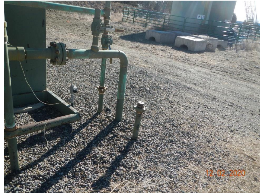
Unused and unmarked flowline riser
