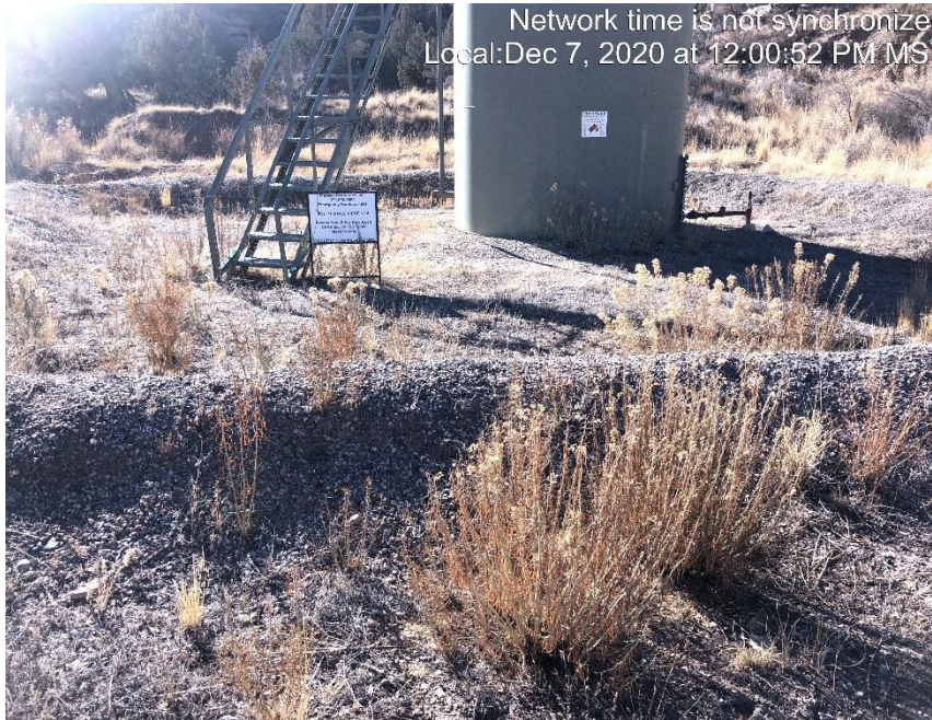
Photo #2411 Secondary containment not adequate weeds and debris inside tank containment.
