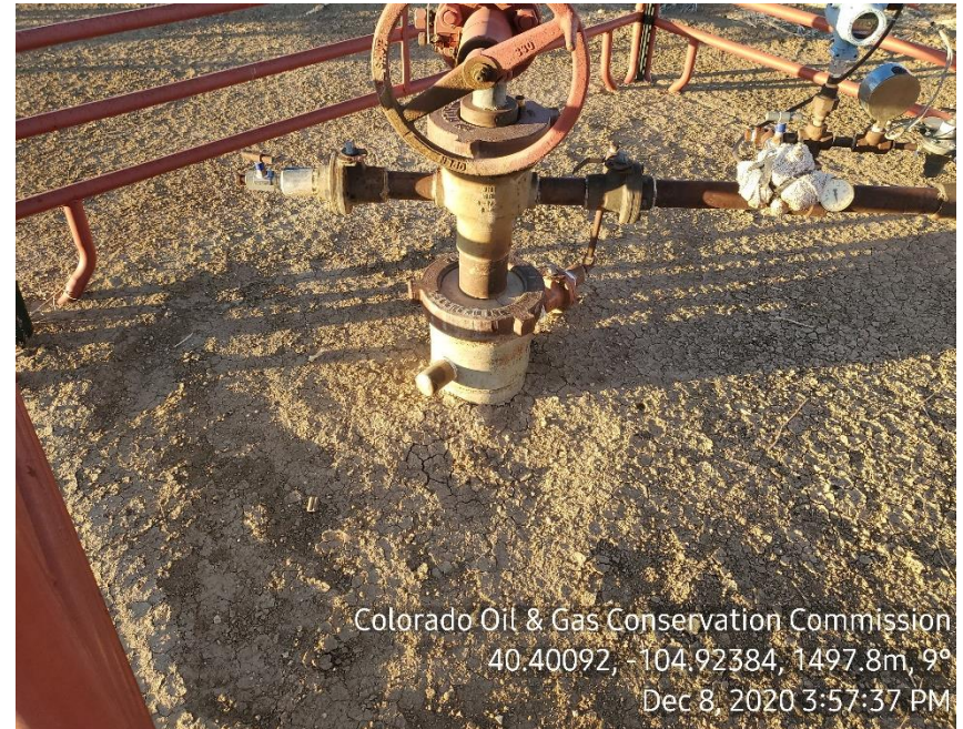
Photo 2: Stained soil removed
