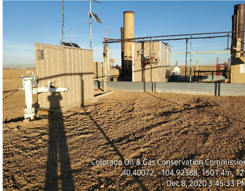
Photo 3: Disconnected gas meter removed
