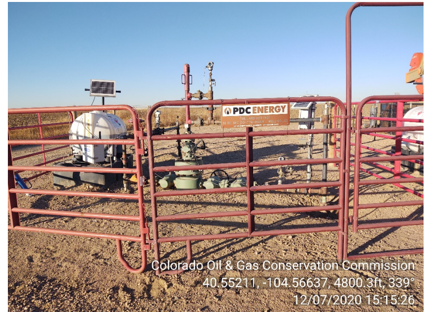
Photo #4 Dillard 20T-401 (05-123-36601) Wellsite Producing | PR Gas lift manifold present (Adjacent to chemical tank)
