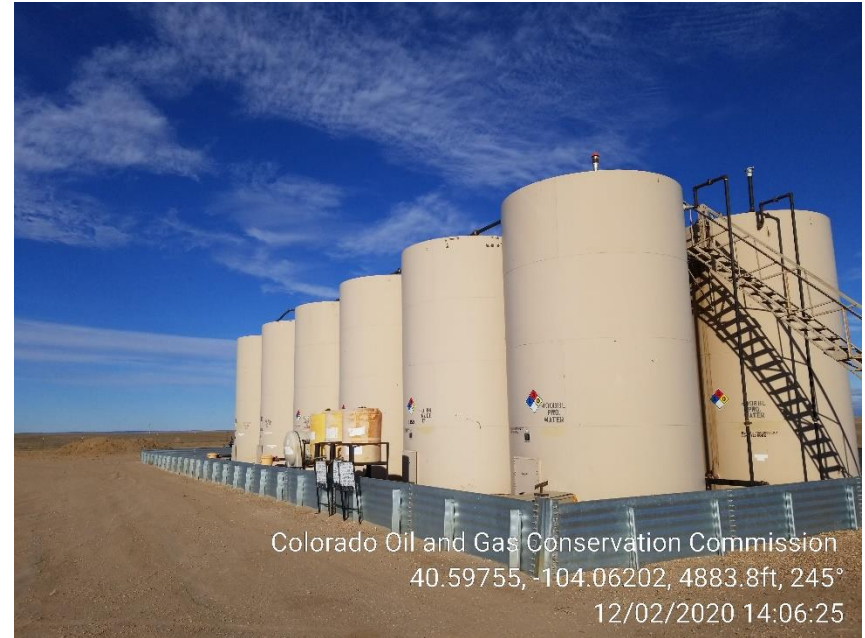
Photo 20 – Tank Battery
