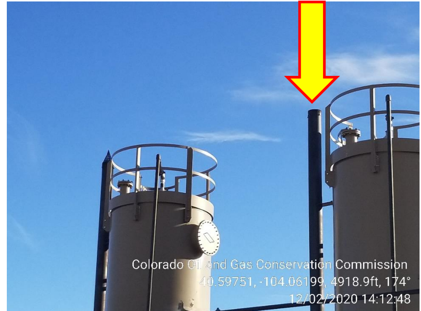
Photo 18 – West Heater Treater appears to be missing Bird Screen Protector
