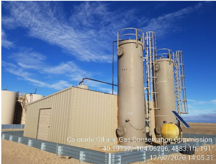
Photo 17 – Heater Treaters
