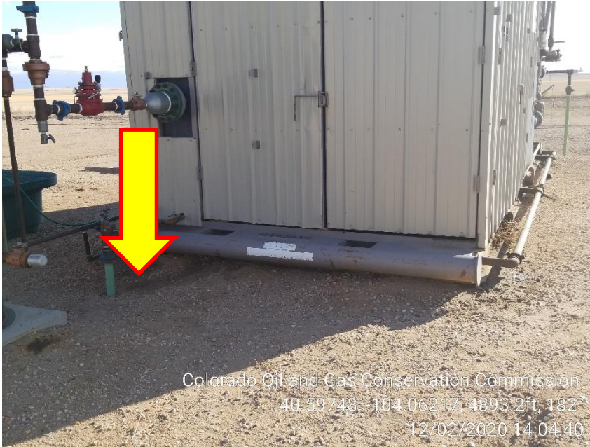
Photo 13 – Stained Soil at Compressor
