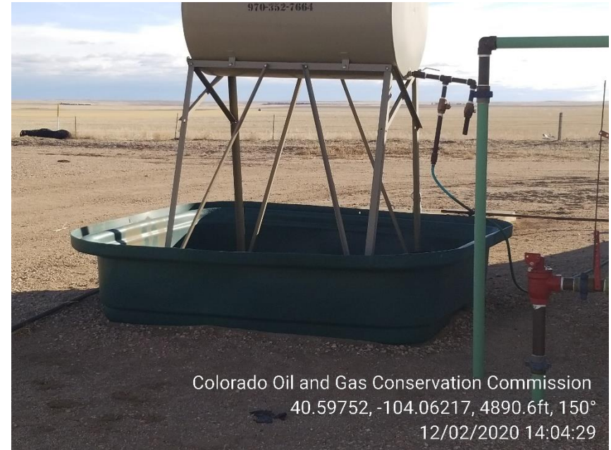
Photo 12 – Day Tank at Compressor missing Wildlife Netting
