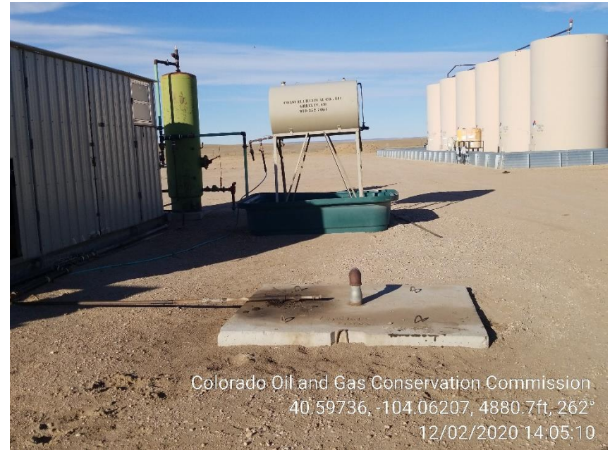
Photo 16 – Drain Vault at Compressor missing Lables – Content, Capacity and NFPA
