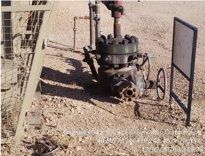
Photo 7 – Stained Soil at 2-3H Wellhead
