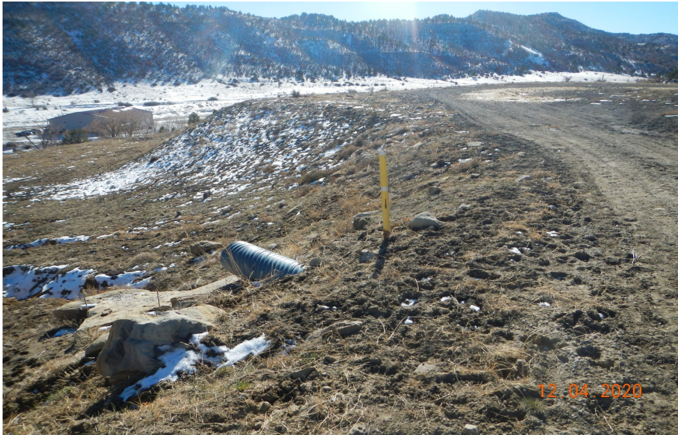
Photo 2. Facing southeast toward the fill slope of the location.
