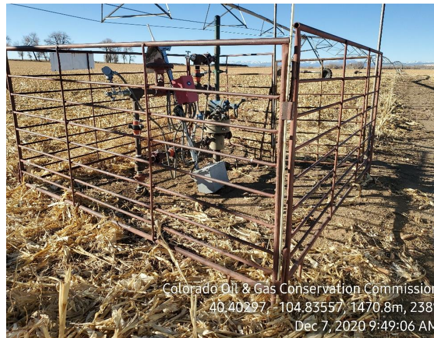
Photo 2: Wellhead; weeds removed
