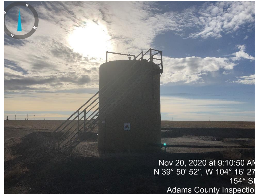
Photo #4 Produced water tank.
