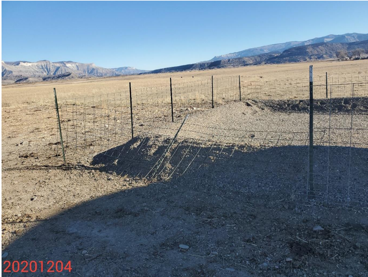
Photo 4: Photo taken from the northwest corner of the tank battery. Photo shows fence panel in disrepair. Livestock access within containment berm evident. Advise maintenance to restrict livestock access to battery and containment BMP.
