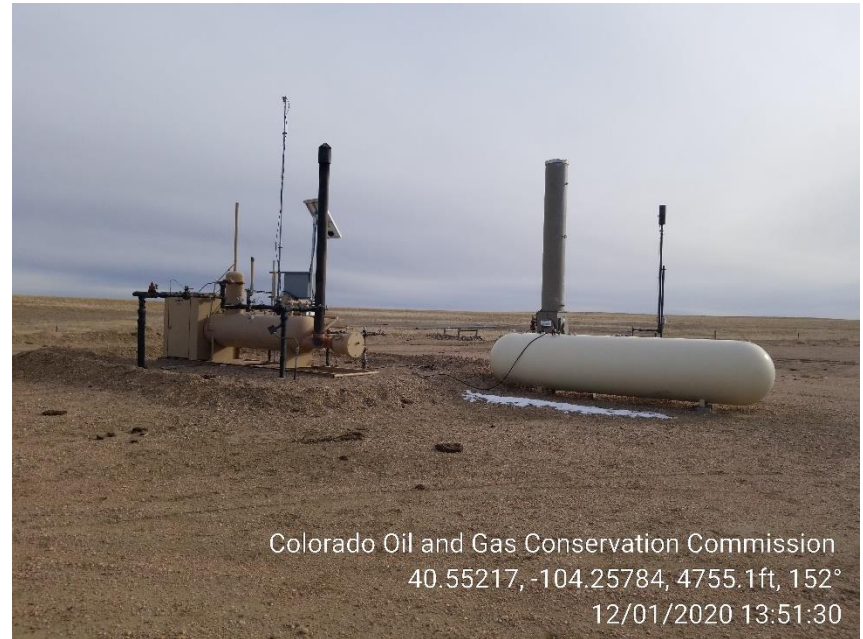
Photo 2 – Separator, ECD and Flare
