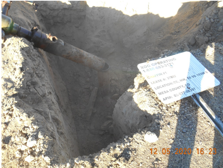
Wellhead / Casing cutoff
