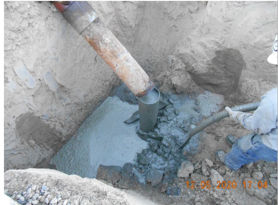
Wellbore topped off with cement
