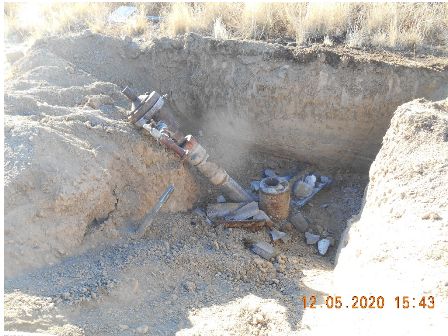
Wellhead / Casing cutoff
