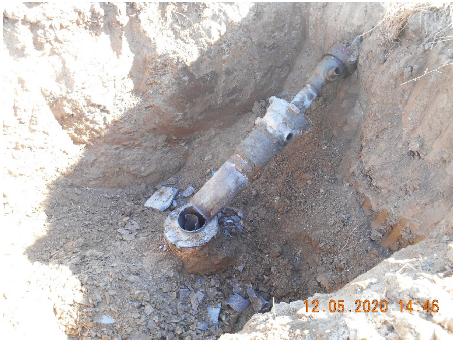
Wellhead / Casing cutoff
