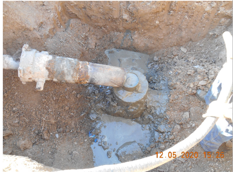
Wellbore topped off with cement
