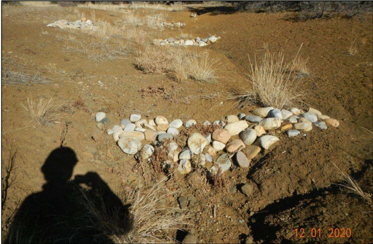
Photo 5. View of erosional channel/diversion in the southeastern project area where cobble BMPs are not adequate. Channeling around cobble, sediment deposition, and further channeling are evident. Canada thistles (approx. 50) observed during previous reclamation inspection are still present.
