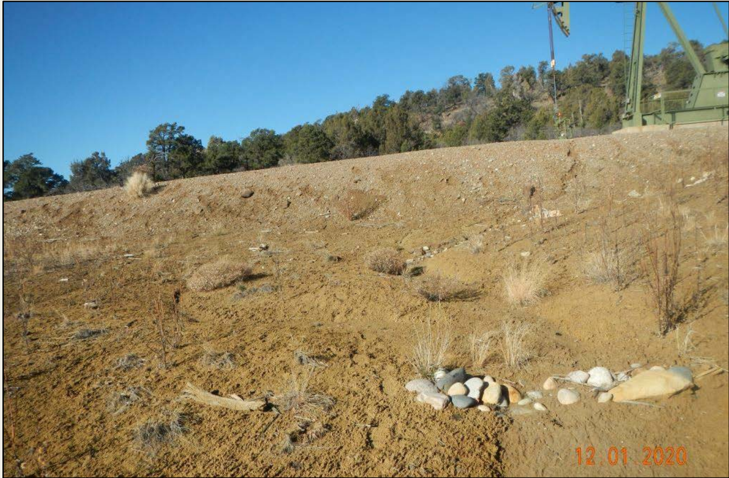
Photo 4. View of area along the southern edge of the well pad where stormwater flows off of the well pad creating erosional channels shown in Photos 3 and 4.
