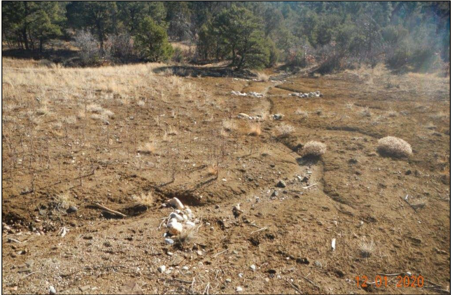
Photo 2. View of erosional channeling in the southern project area. Cobble in channels is not an adequate BMP. Bare soils in southern portions are not stabilized.
