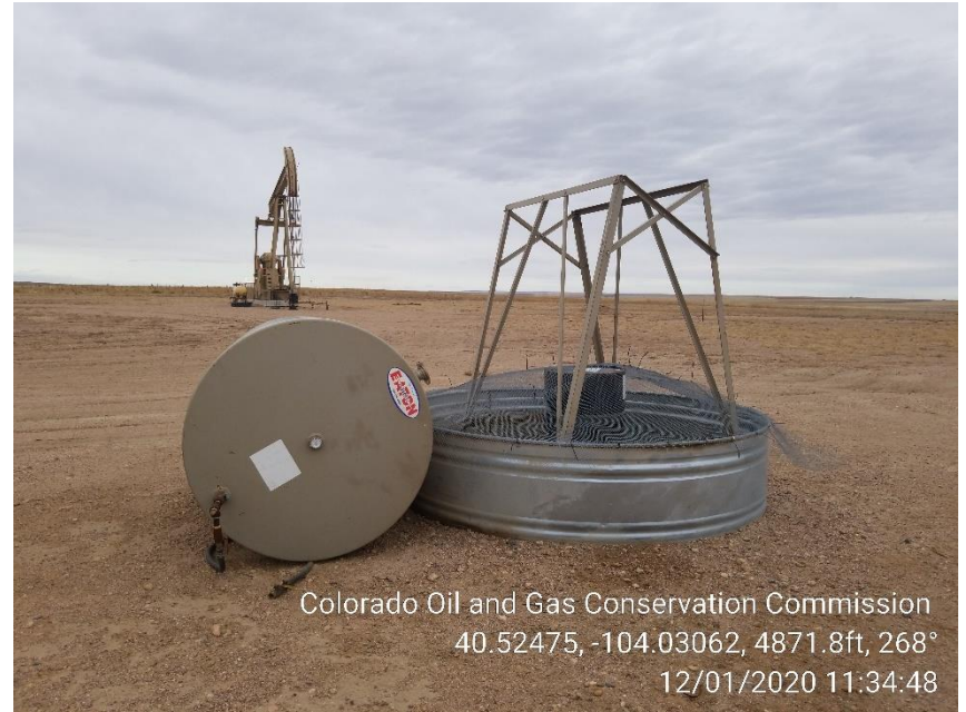
Photo 14 – Stained Soil cleaned and Wildlife netting installed
