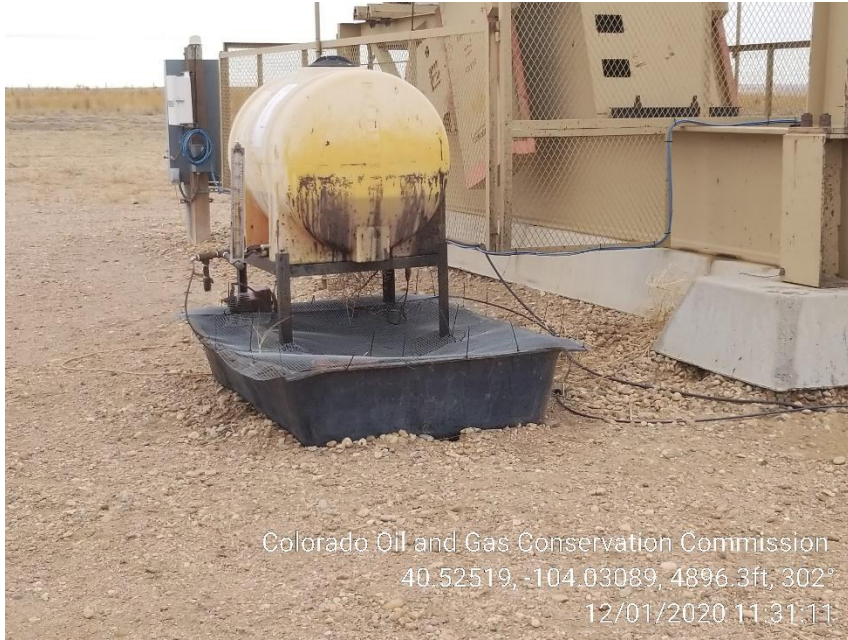
Photo 13 – Stained Soil cleaned and Wildlife netting installed
