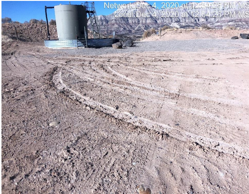
Photo #2402 Sediment is being transported off of location due to tracking and lack of stabilization.
