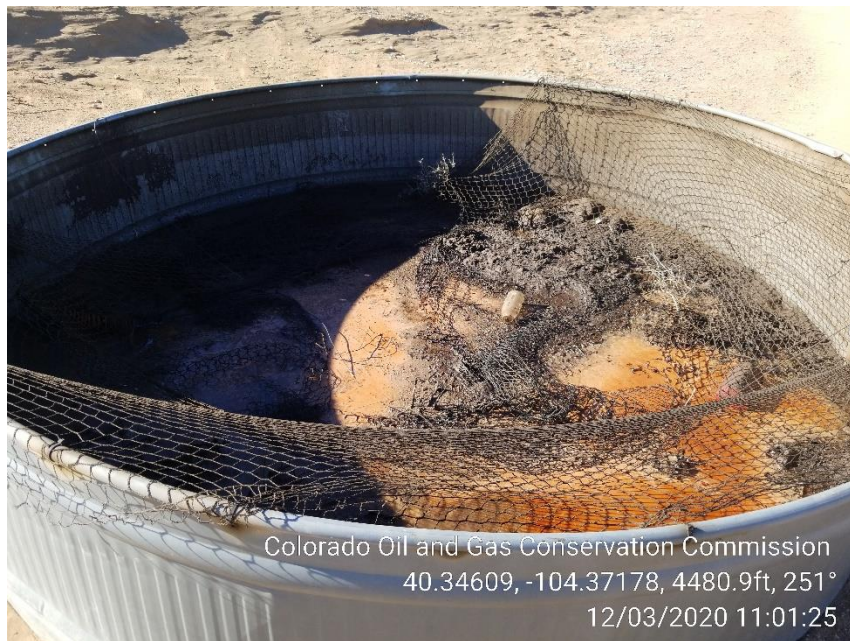
Photo 15 – Containment – Oily Waste and Wildlife Netting in disrepair
