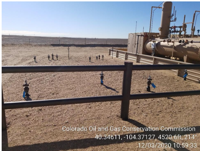
Photo 7 – Risers at Separators now Marked
