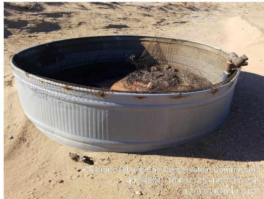
Photo 16 – Containment – Oily Waste and Wildlife Netting in disrepair
