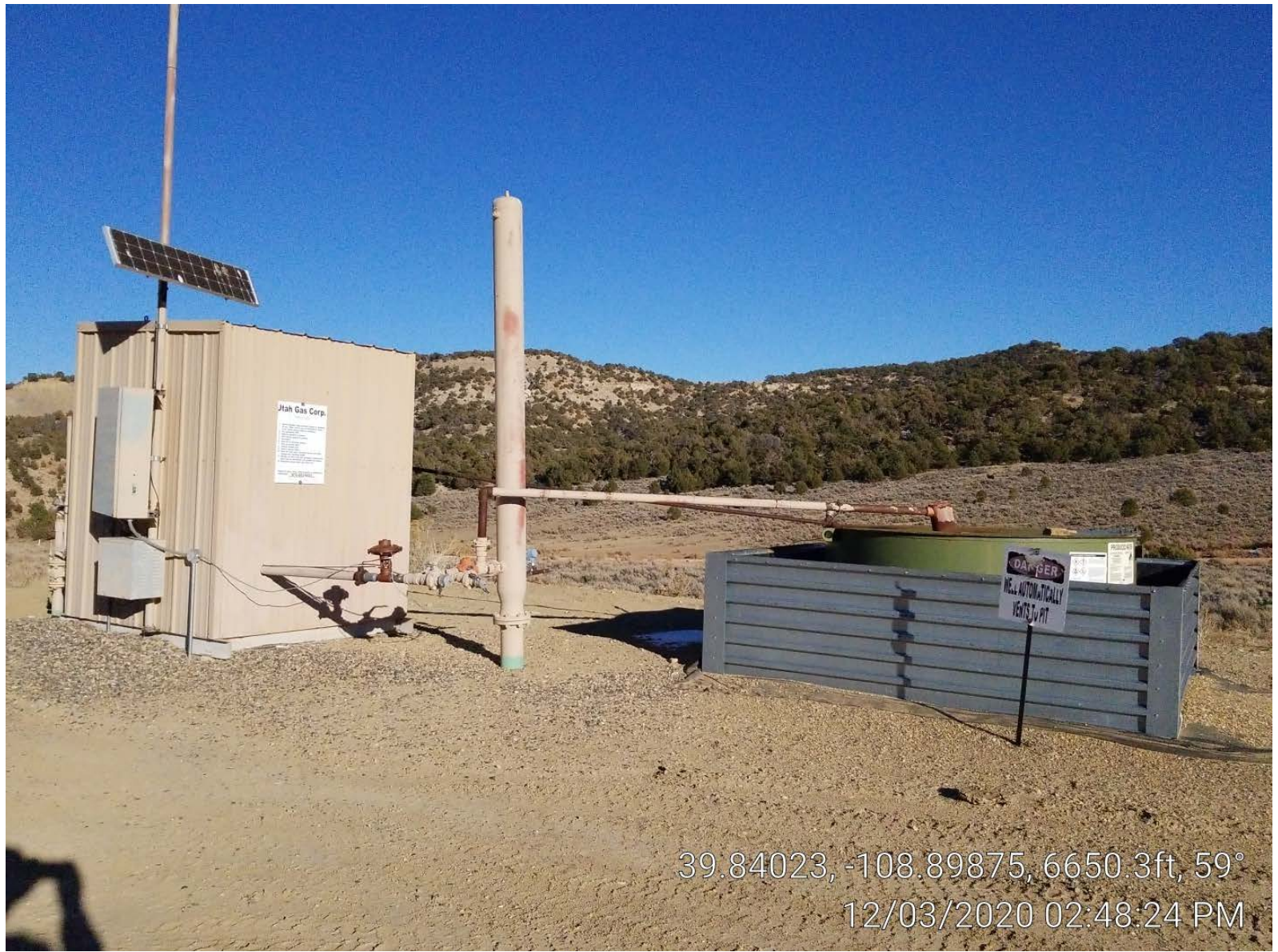
Photo 2. Meter building & tank.
