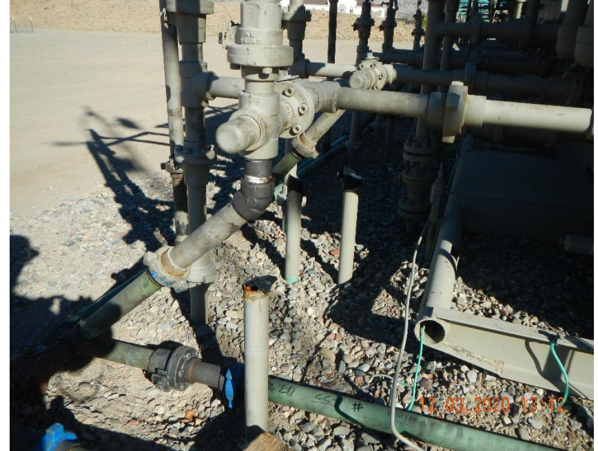
Unused 2" flow line risers in front of separators.
