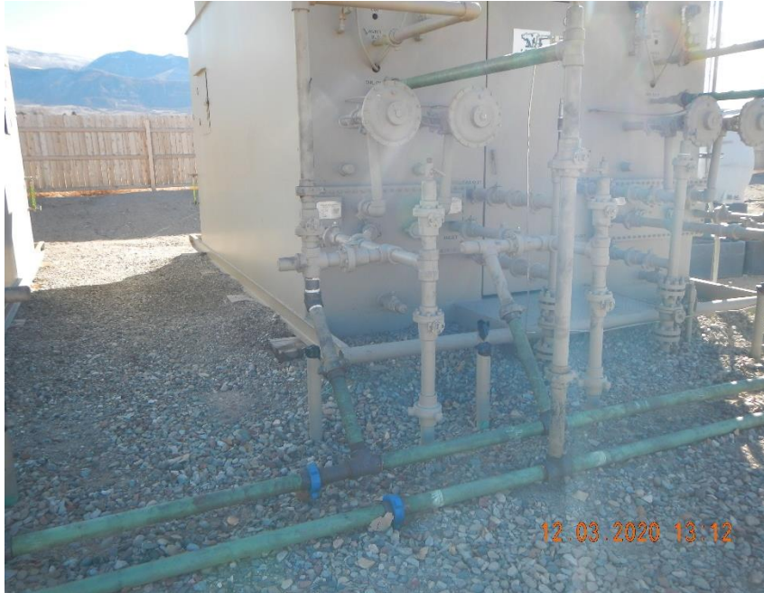
Unused 2" flow line risers in front of separators.
