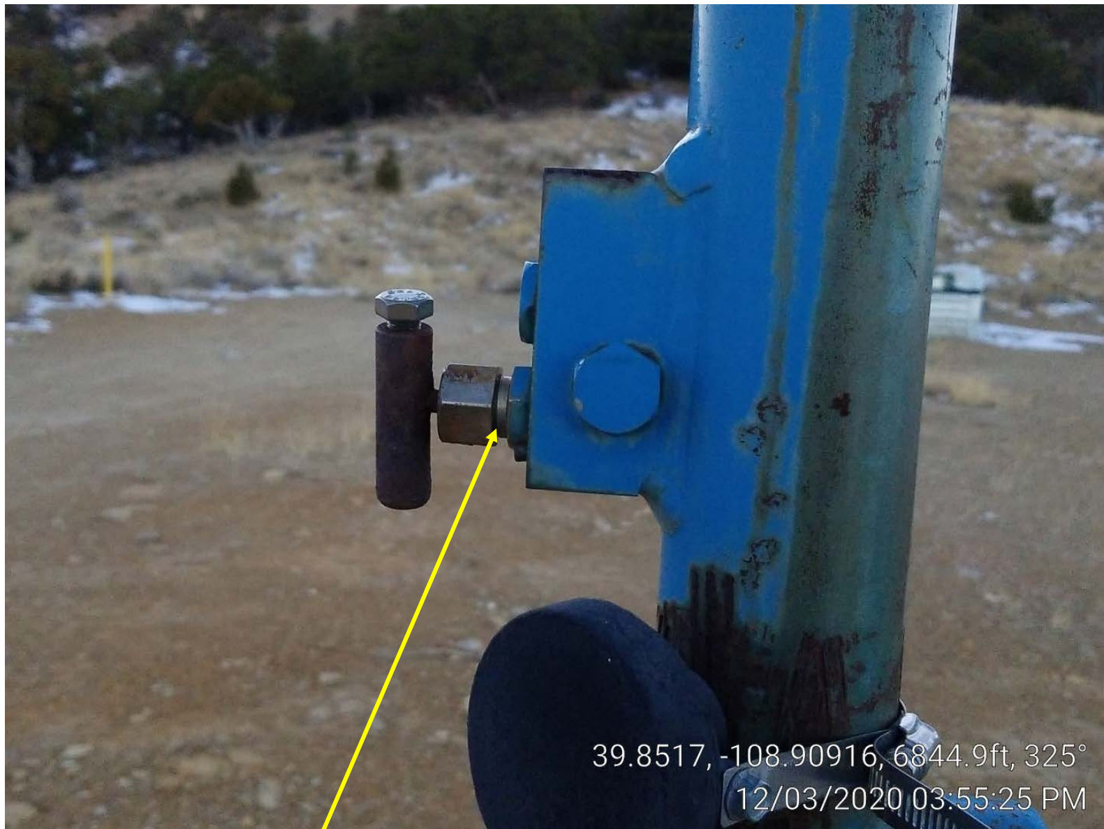
Photo 3. Gas leak.
