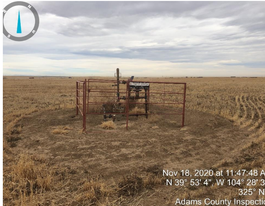
Photo #3 Well Head.
