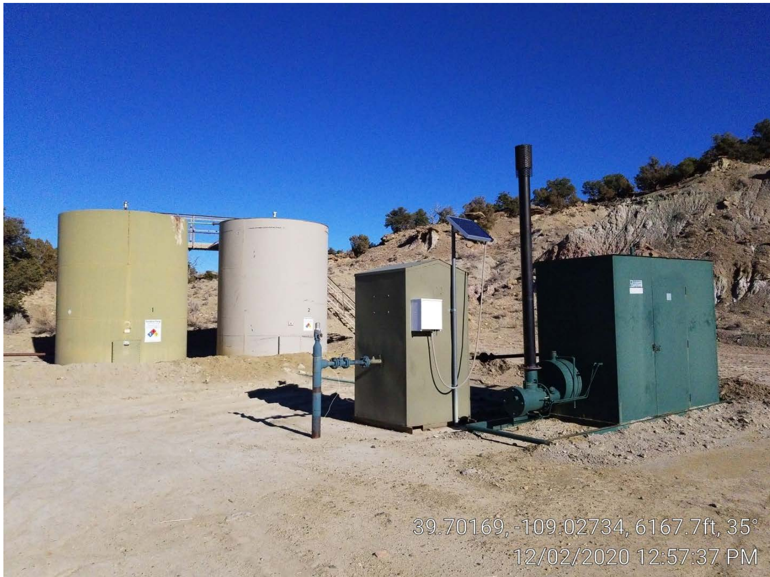
Photo 2. Tanks, meter building, separator.
