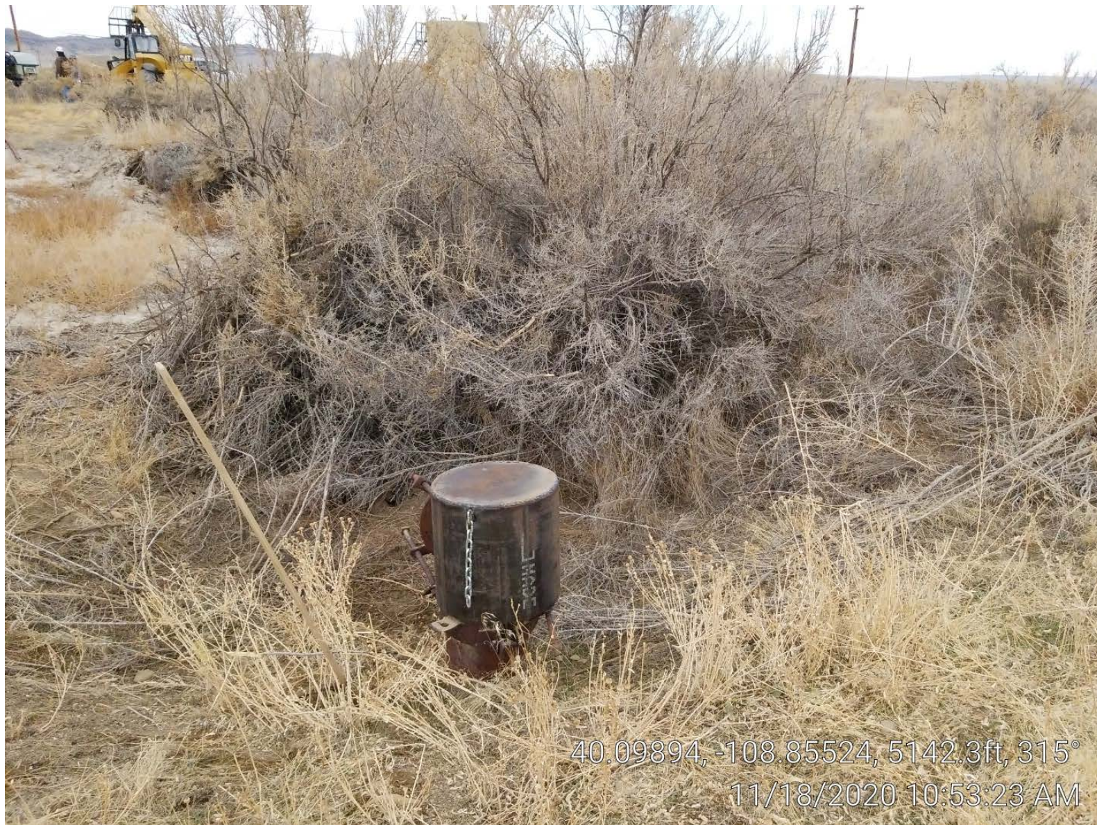
Photo 1. Well before plugged with temporary hood cover.
