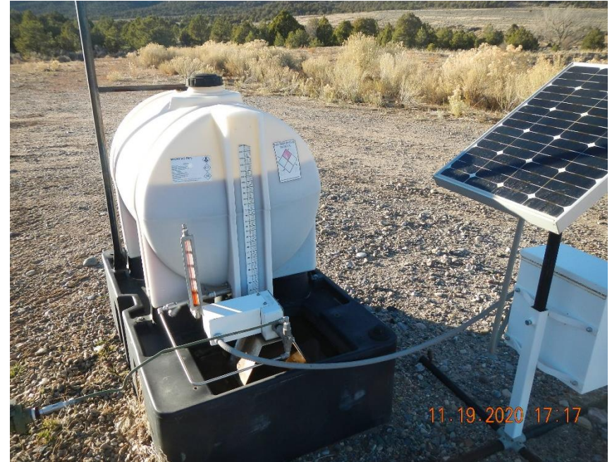
Chemical injection system with secondary containment.
