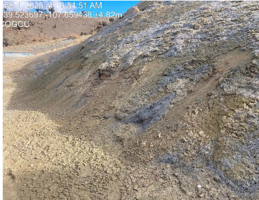
Lack of stabilization/erosion
