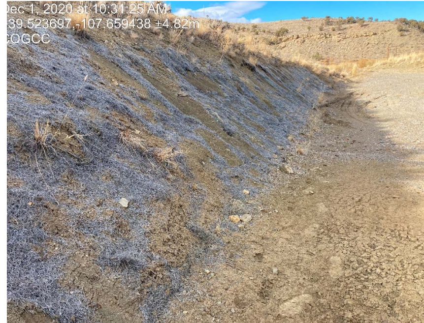
Lack of stabilization/erosion
